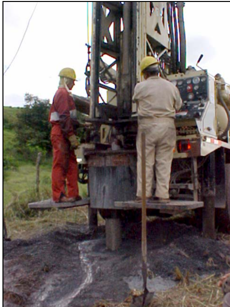
Fig. 5.2a: Photo of a well being drilled. Two well perforators are working with the drilling. Soil, rock material and fluid come up from the drill hole.
