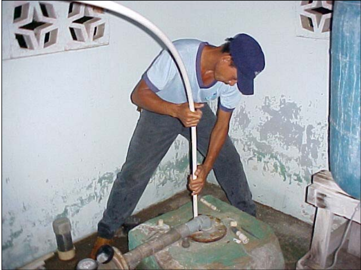
Fig. 6.2.4b: Photo of well operator Luis Valdez, IDAAN, taking out the plastic tube in well 1 (IDAAN B1) in Pesé so that measurements can be done.
