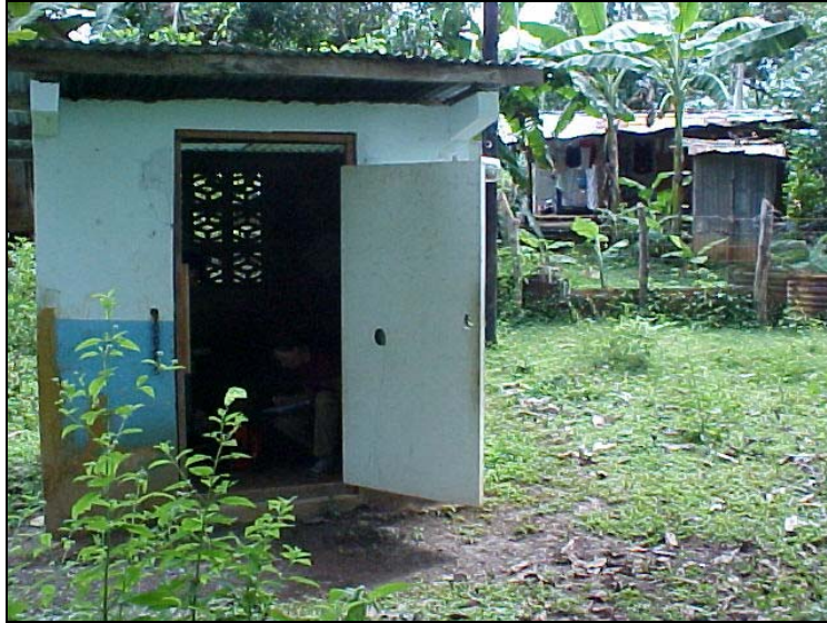
Fig 6.7.1a: Photo of a well-house painted in white and blue close to an outside lavatory in the outskirts of Pesé.
