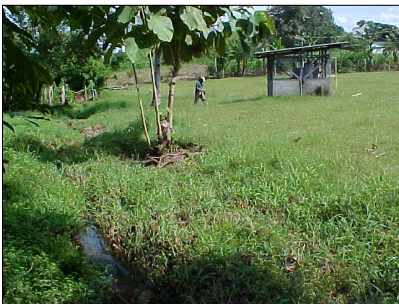
7. A pump house for a well in Sabana Grande
